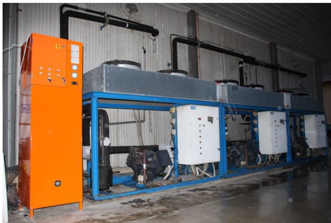
Figure 4: Pilot Plant – Cooling Power 30kW
